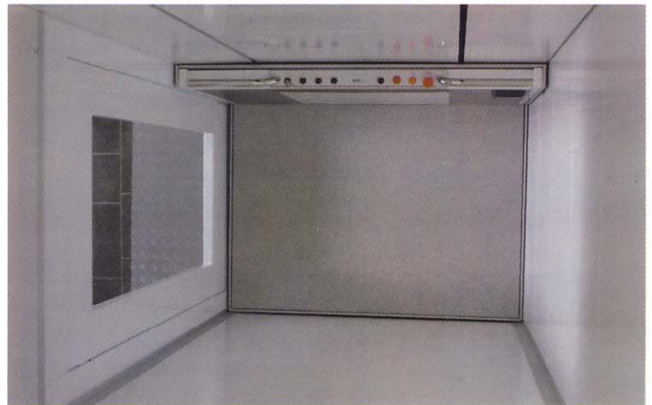
Platform and panel from above.
