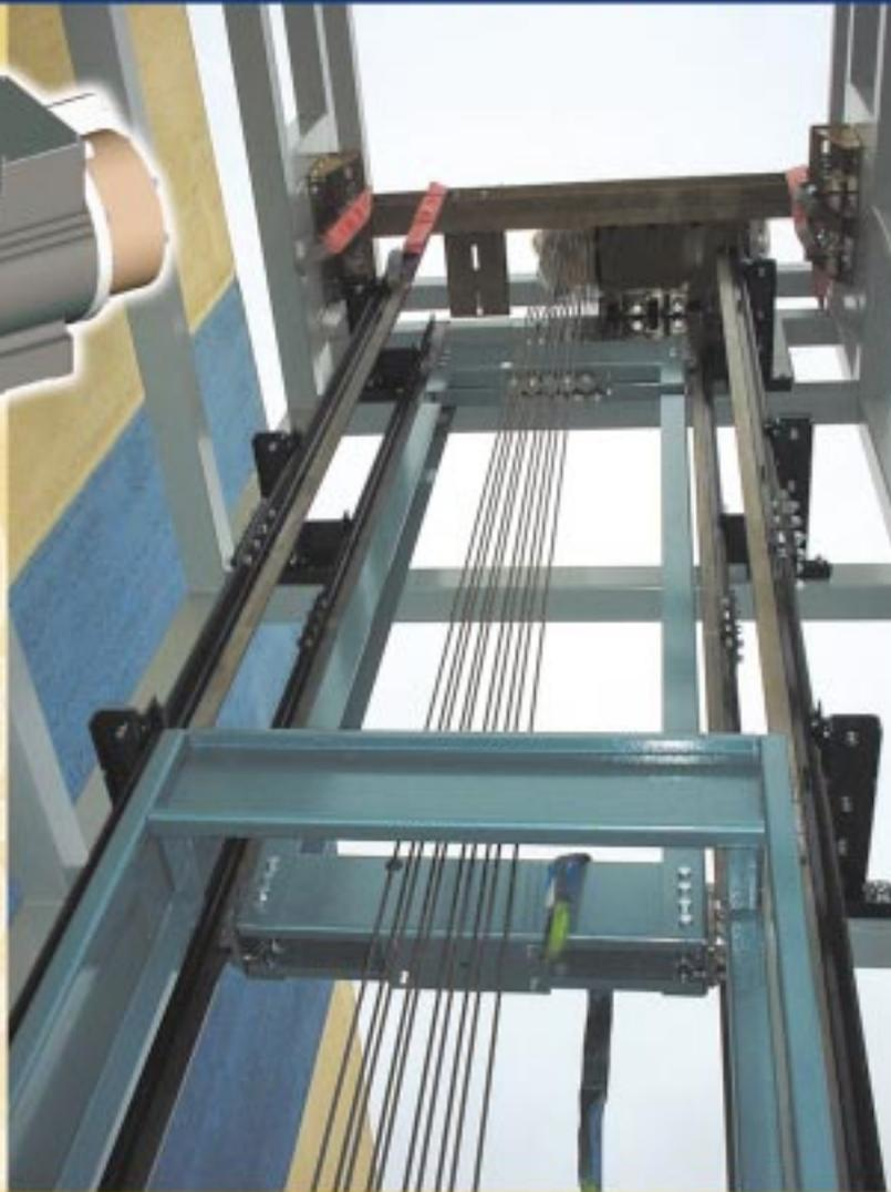
The Machine Room-Less Lift, specially designed for high - rise buildings and heavy loads
